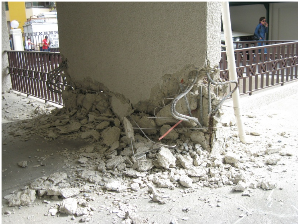
Figure 5-7 Crushing and bar buckling in the transverse shear wall on Line 1 resulting in significant differential vertical displacement (photo courtesy of Patricio Bonelli).
