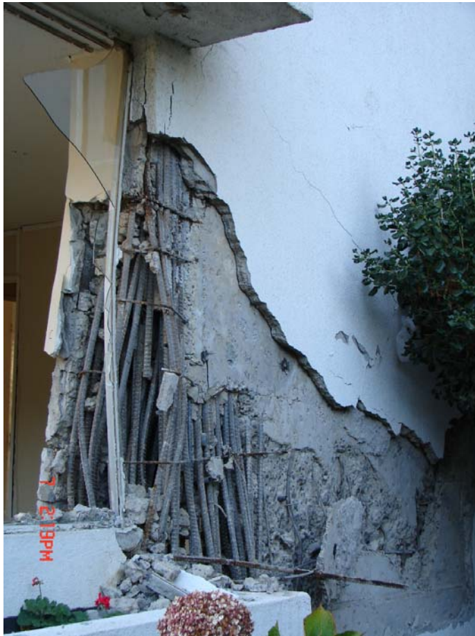
Figure 2-7 Damage to typical unconfined shear wall boundary zone observed in the 2010 Maule earthquake (photo courtesy of ASCE).
