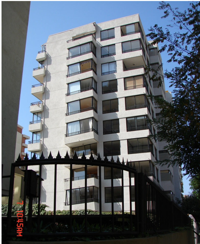
Figure 5-3 Transverse elevation of the case study building showing differential vertical displacements following the 2010 Maule earthquake (photo courtesy of Patricio Bonelli).
