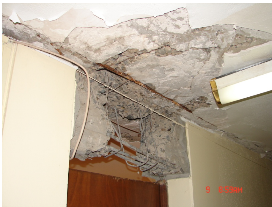
Figure 2-5 Shallow lintel showing nominal reinforcement and lack of confinement in a residential building that was damaged in the 2010 Maule earthquake (photo courtesy of ASCE).
