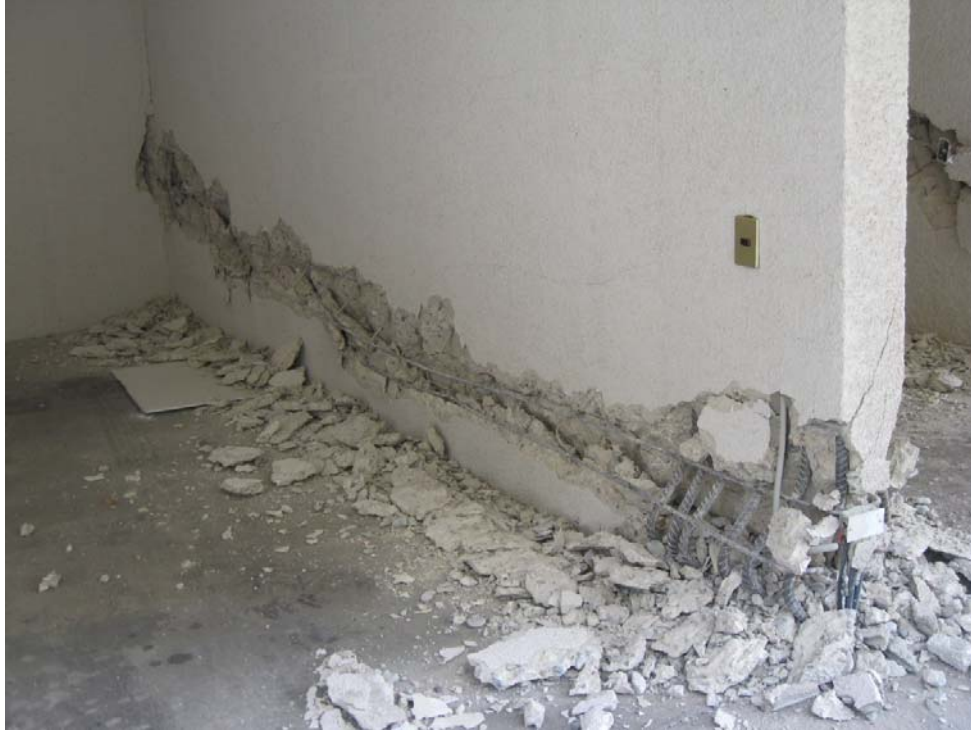
Figure 5-6 Cracking, spalling, crushing, and bar buckling in the transverse shear wall on Line 5 (photo courtesy of Patricio Bonelli).
